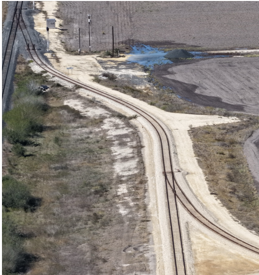
Rail Switch & Lead Track Connection
